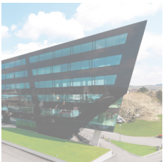
MP09 office building, Graz, AT
